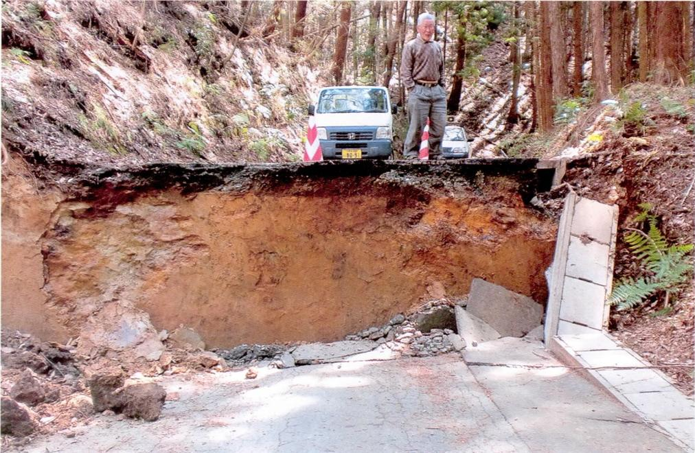
There are multiple faults running through underground Tabito machi. The April aftershocks created a level difference of 2 metres in many places.
