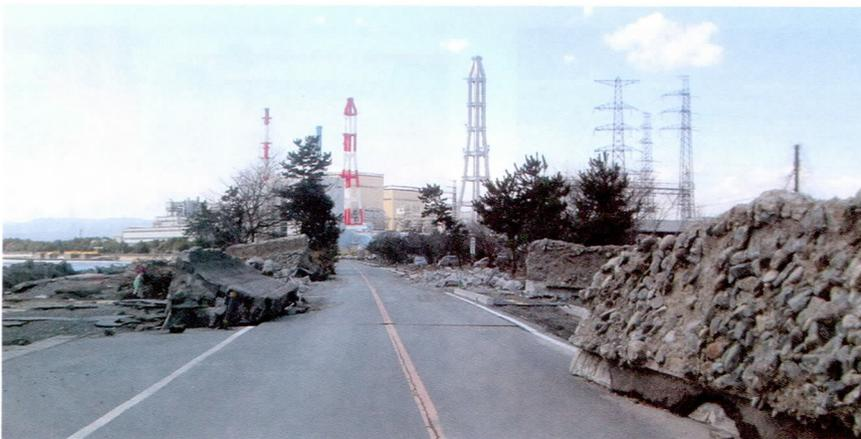
Breakwaters were swept over the street by the tsunami in Iwama district. Chimney shown in the photo is from the Nakoso Power Plant, Joban Joint Power Co., Ltd. The power plant was also damaged by the tsunami, but restored their main generators 8 & 9, and then they also recovered the generators 6 & 7 which were stopped, and supplied electricity to TEPCO and Tohoku Electric Power Co.
