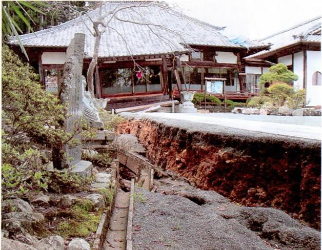
The April 11 & 12 severe aftershock woke up the long-sleeping fault. Cracks in Kentokuji Temple in Joban Fujiwara machi.
