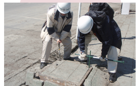
Investigation into damage to sewers (Matsushima, Miyagi Prefecture, Mar. 24)
