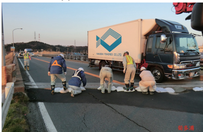
Running restoration work of bumps on Route6 (Apr.12)
